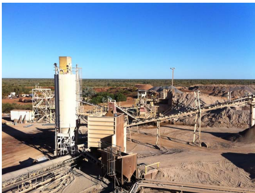
Figure 6: Western Tanami Operation Plant
